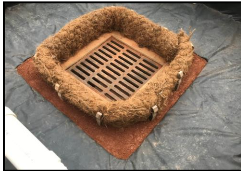
Test Setup and Installation Zone around 24-in x 24-in Inlet
